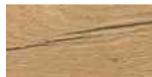
1111 HALIFAX CRACK OAK
